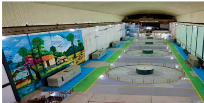
Fig. 9 Pump House equipped with 4x134.4 MW Pumps
