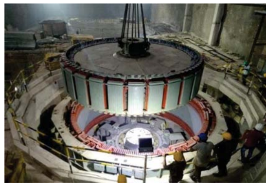
Fig. 8 Lowering of Rotor Assembly of 125 MW Pump
