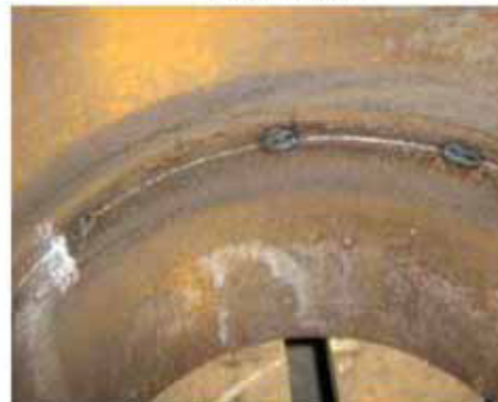
Fig No. 18: Aligned pipes with tack welds
