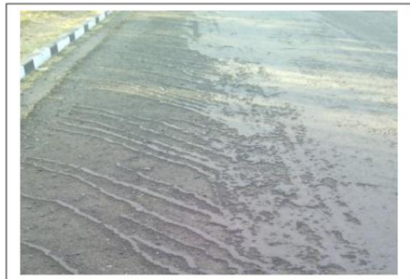
Image No 6 : Emulsion Sprayed portion is Safe and firm.
