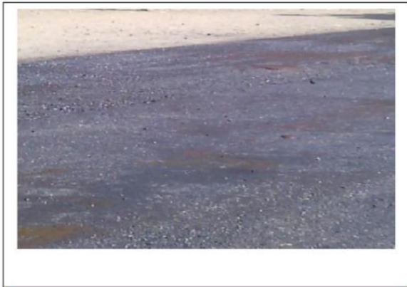
Image No 1 :Emulsion & Sand Sprinkling
