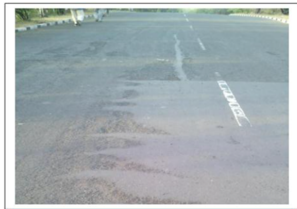
Image No 5 : Emulsion Sprayed portion is Safe and firm.
