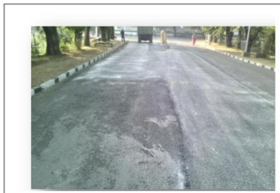
Image No 10 :Patch work done in portion where preventive measures has not done.
