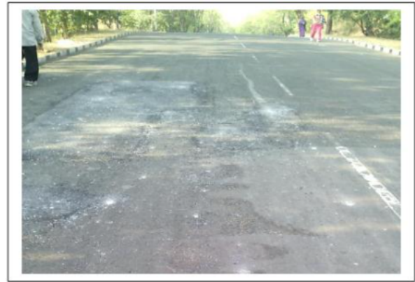
Image No 4 : In Dec 2014 Patch repair is being required & done. Latitude 23.138357 Longitude 79.912673.
