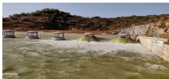
Fig. 5 Delivery Reservoir: Package 6
