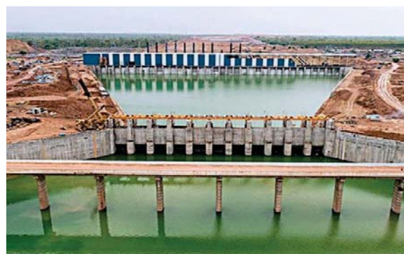
Fig. 4 Overview of the Medigadda pump house [4].
