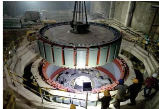
Fig. 8 Lowering of Rotor Assembly of 125 MW Pump
