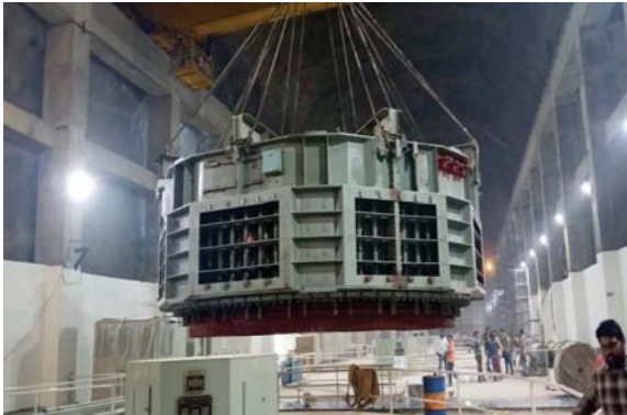
Fig. 7 Lowering of 200 t Stator Assembly of 116 MW Pump
