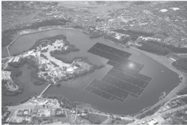
Fig. 5: Floating solar panels
