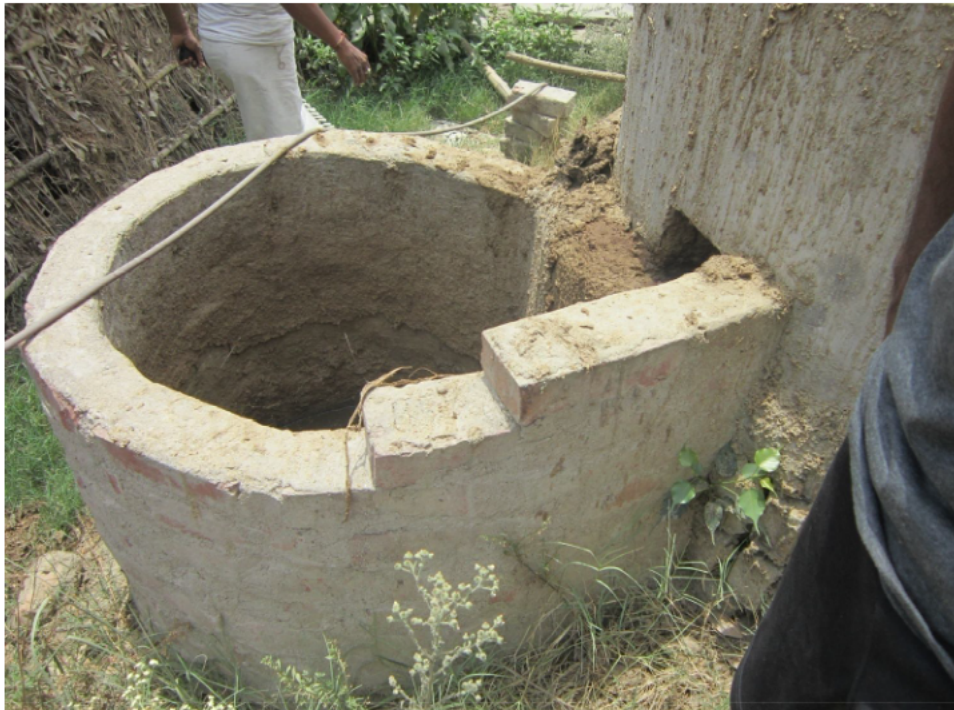
Fig. 2: A Biogas plant installed by Mr. Jay Shankar, Gram- Taiteri, District –Begu Sarai, Bihar
