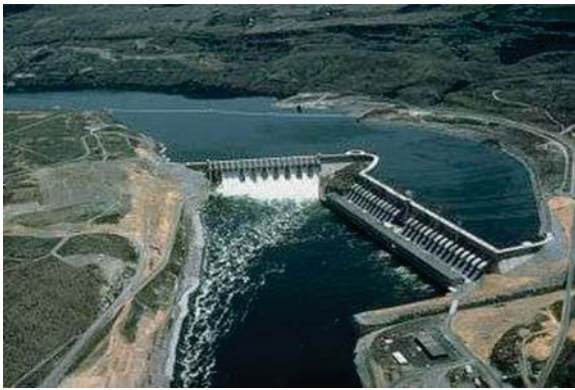
Fig. 2 Chief Joseph, the world's largest run-of-the-river hydroelectric power project [5].
