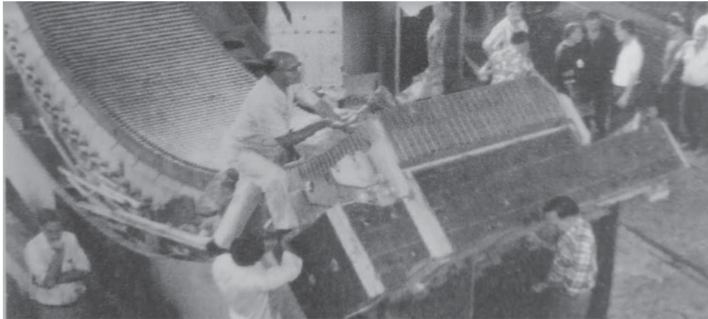
Fig. 5 Repair of stator winding segment at site
