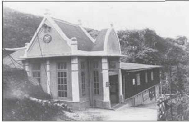
Fig.3 Hydro power station at Darjeeling [5]
