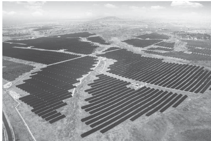
Fig. 4 Largest solar power plant of the world at Bhadla, Rajasthan [7]
