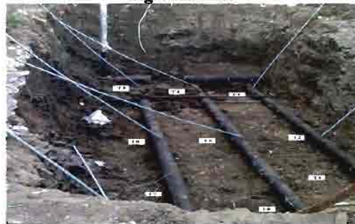
Fig. 8 Tube Placed Inside Earth
